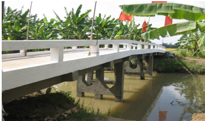
Figure 2. The new bridge
