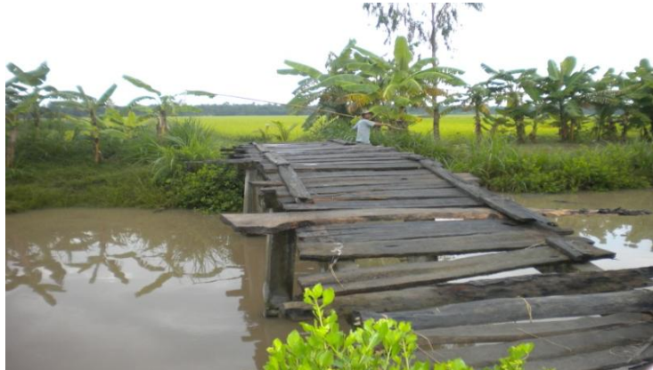
The wooden bridge
